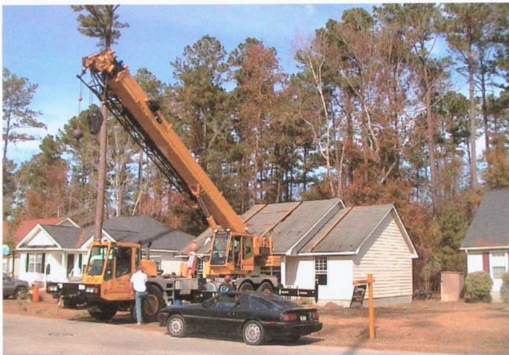
Figure 3. Crane Used to Conduct Uplift Tests with 3656 Eagle Trace in Background.
