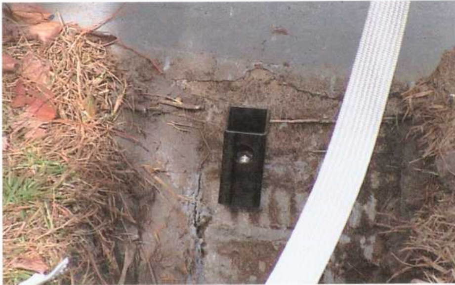
Figure 1. Anchor Bracket Attached to Foundation Using Epoxy Grouted Stainless Steel Anchor Bolt.
