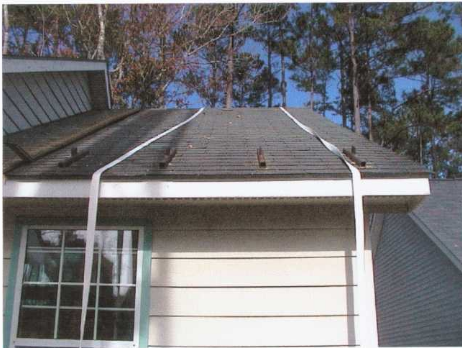
Figure 2. Orage Corporation Over the Roof Straps on 3656 Eagle Trace.
